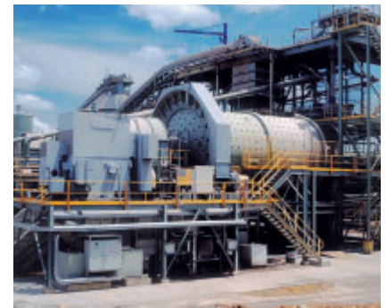
Bearing arrangements in comminution and processing plant
