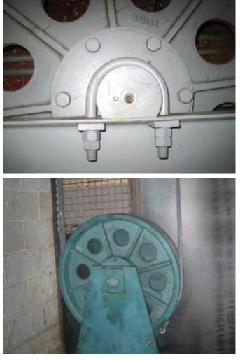
Fig. 15 AP bearings shown on typical elevator sheave application
