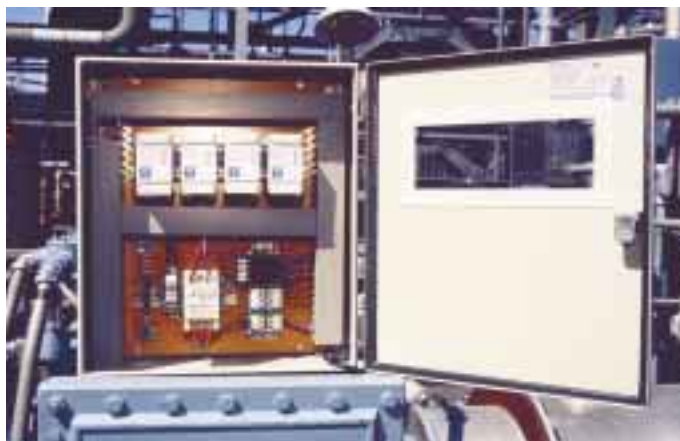
Electronic cabinet with built-in MCM™ units
